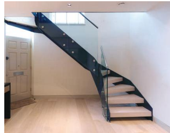
7 'Project' Broadlands Construction, Mayfair 2014.
